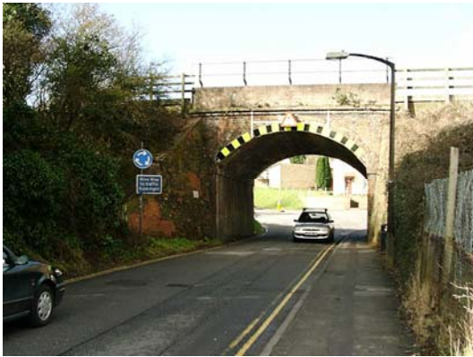
Laverstock Road railway arch (looking West)
