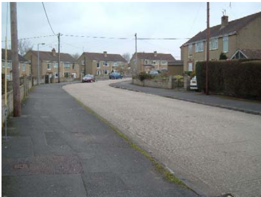
Napier Crescent, looking North
