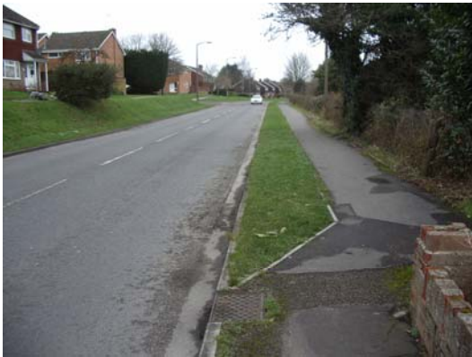
Manor Farm Road footpath, east side, looking North
